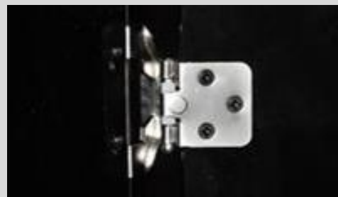
Self closing hinges to prevent wood-on-wood contact.
