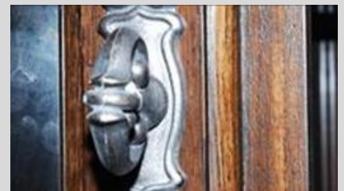
Clear-coated to protect from water, finger oils and oxidation.
