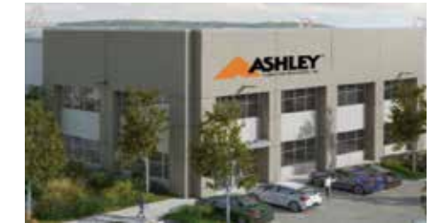
Spanaway, WA: Opening in 2021 1,000,000 sq. ft. | 92,093 sq. mt. | 23 acres under roof
